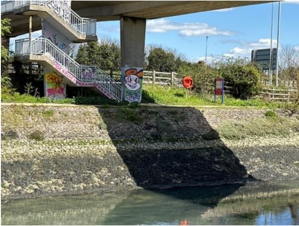
Photograph Z.7.2. : Portsbridge Creek with PRE and Signage
