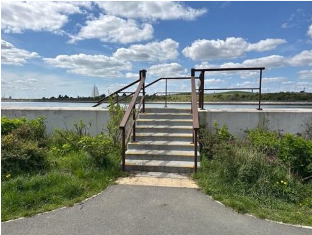
Photograph Z.8.2. Egress Access to Tipner Lake
