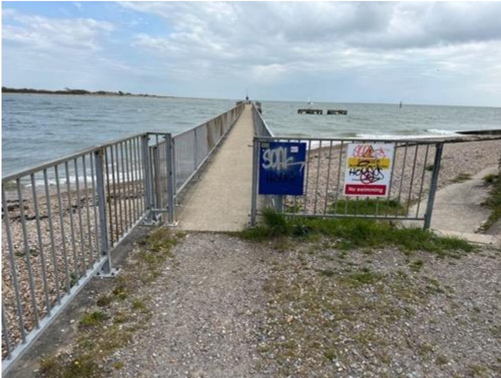
Photograph Z.4.2 Outfall and Signage
