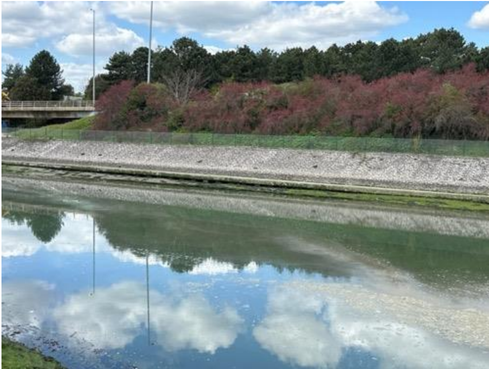
Photograph Z.8.4. Hard Engineered Edge Protection
