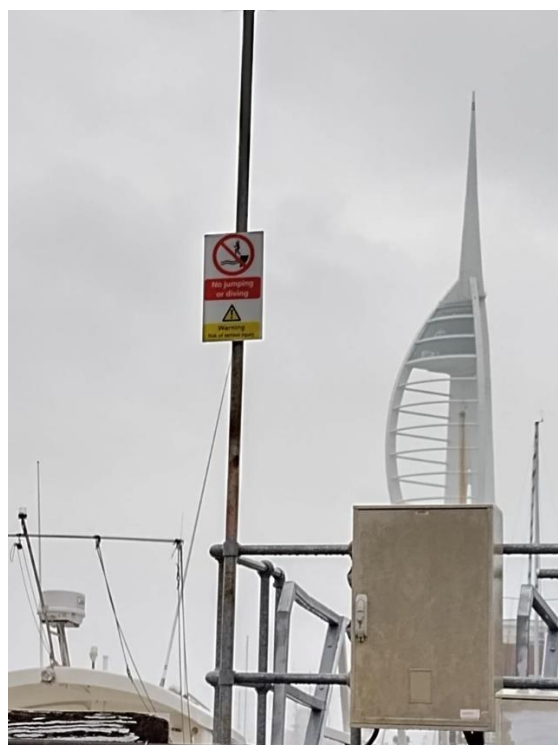
Picture Z13.5 No Jumping signage - Camber
